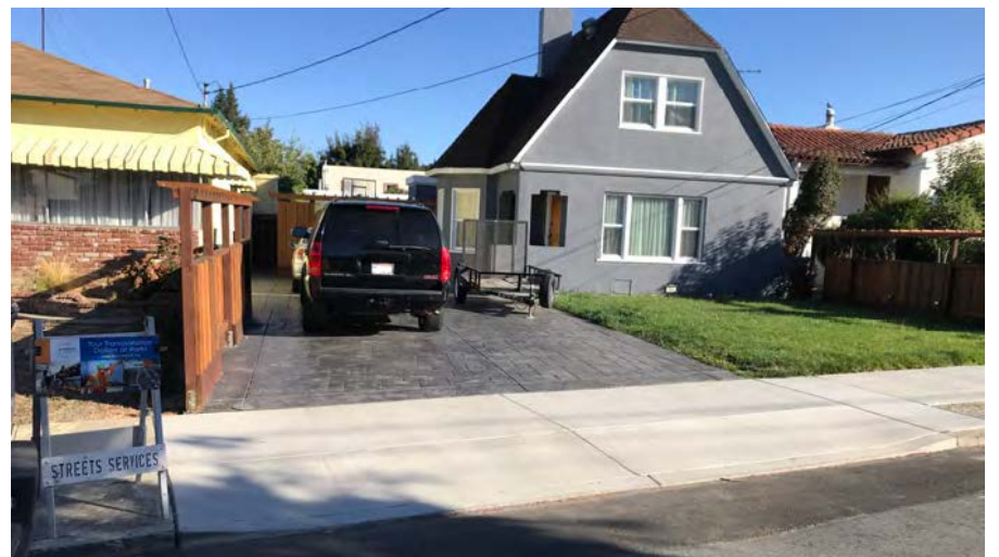
Driveway / Sidewalk Repair
