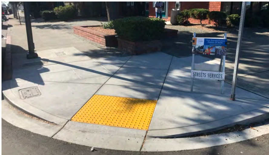
Curb Ramp Construction
